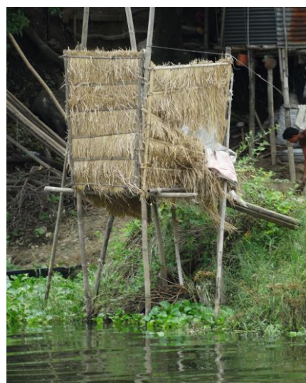
Pictured: At left , an offset pit latrine discharging into the household pond. At right , a ‘hanging latrine empties directly into the canal below.
