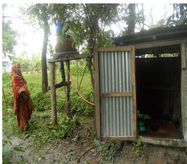
Rudimentary running water supply
